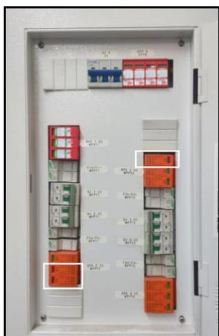
Fig. 10. Negative and ground pole of DPS 2 and actuated positive pole of DPS 3 of Inverter 2.
