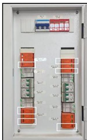
Figure 8. Actuated negative pole of DPS 1 and 4, actuated positive and negative poles of DPS 2 and 3 of Inverter 1.
