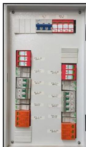
Figure 9. DC protection boxes after changing the SPDs of Inverter 1.
