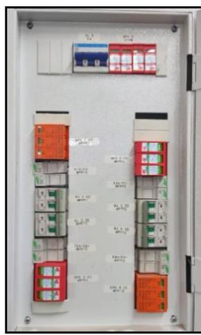
Figure 11. DC protection boxes after exchanging the SPDs of Inverter 2.
